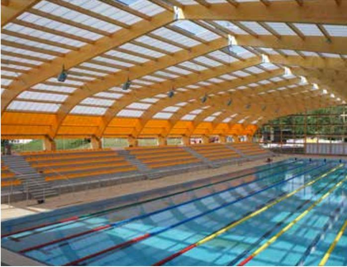
BDL® is a system of standing seam modular panels used to create vertical and sloped glazing. It is suited for a range of applications from curved skylights to interiors. Thanks to its wide variety of accessories, the system is complete, versatile, lightweight, and easy to install.
